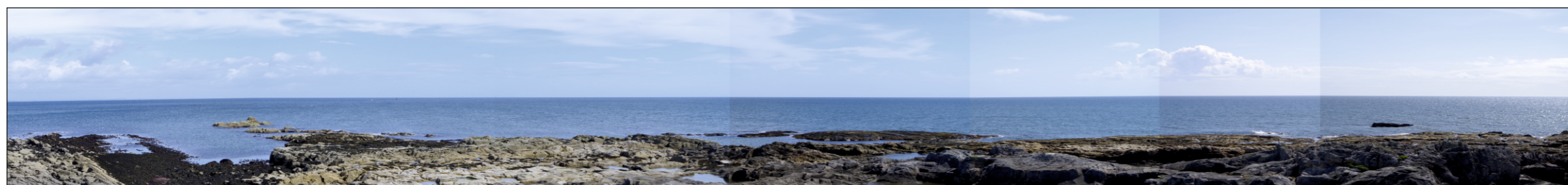
A panorama facing east towards the Offshore Wind Farm from Crail Airfield, pillbox, Foreland Head (SM6461)
