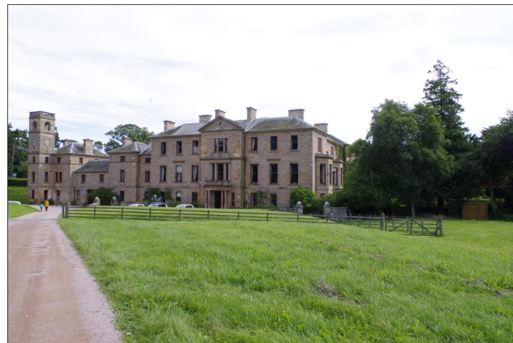
The restricted view at Cambo Estate (GDL00344) House, facing north east
