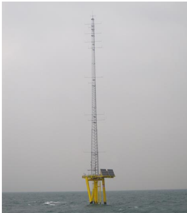
Illustration 4.13: Met mast at Hornsea offshore wind farm (Source: SMart Wind)
