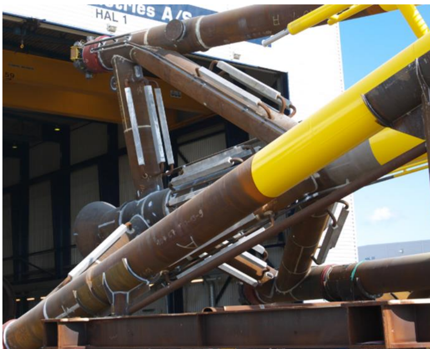
Illustration 4.2: Anodes affixed to jacket members (source: Keystone)
