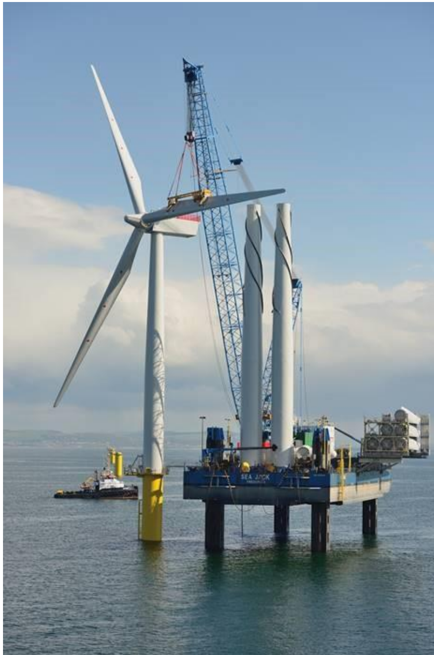
Illustration 4.12: Wind turbine single blade installation (Source: Siemens Gamesa)
