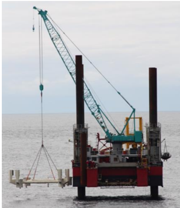
Illustration 4.5: Jack-up barge installing seabed template (source: Fugro Seacore)
