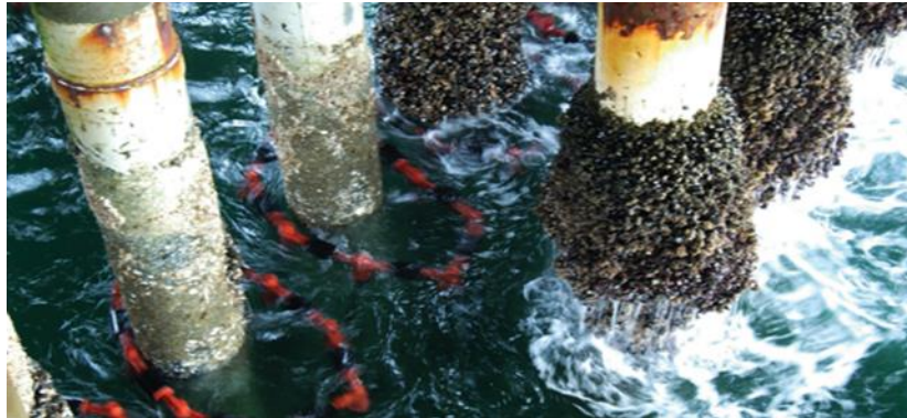
Illustration 4.22: Marine growth prevention solutions (Source: FoundOcean Ltd)
